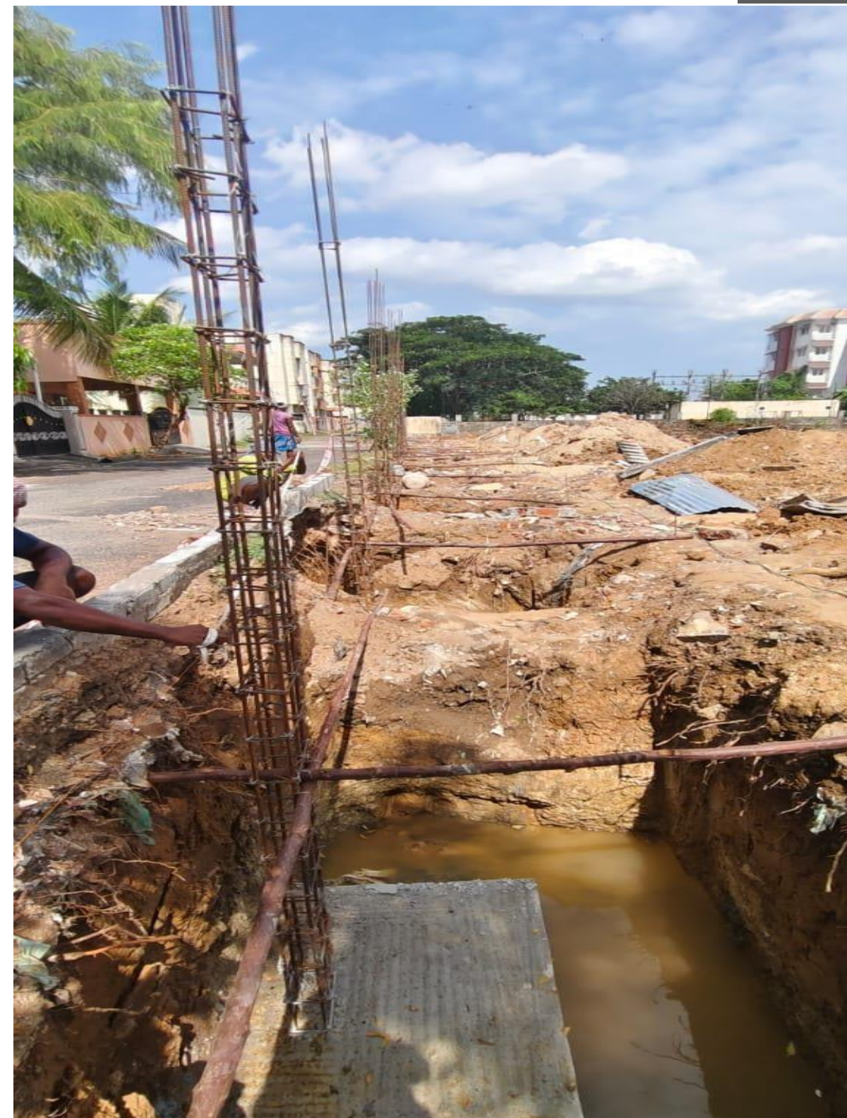
NORTH SIDE COMPOUND WALL FOOTING CONCRETE WORK IN PROGRESS
