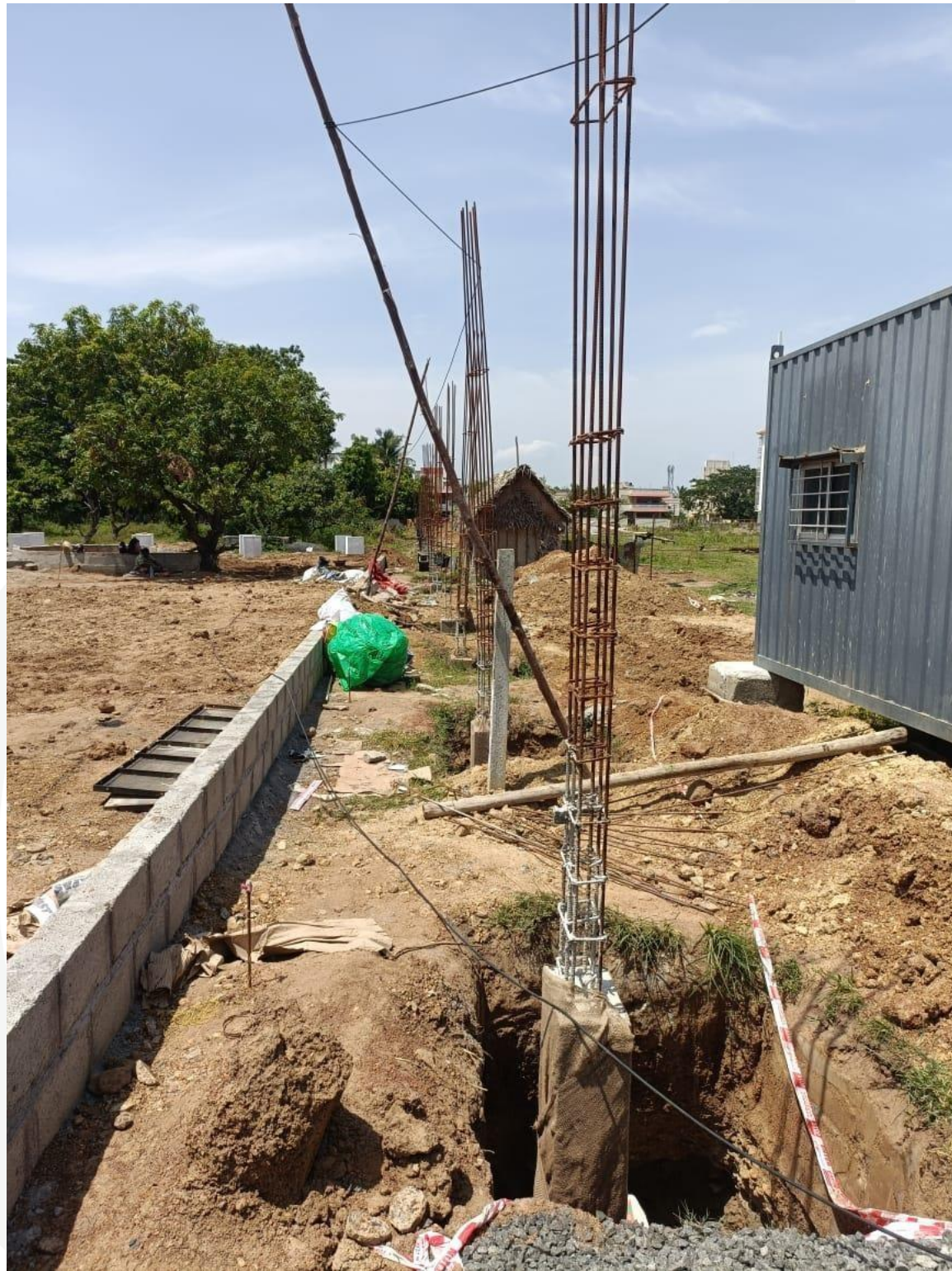
WEST SIDE COMPOUND WALL FOOTING & COLUMN CONCRETE WORK IN PROGRESS
