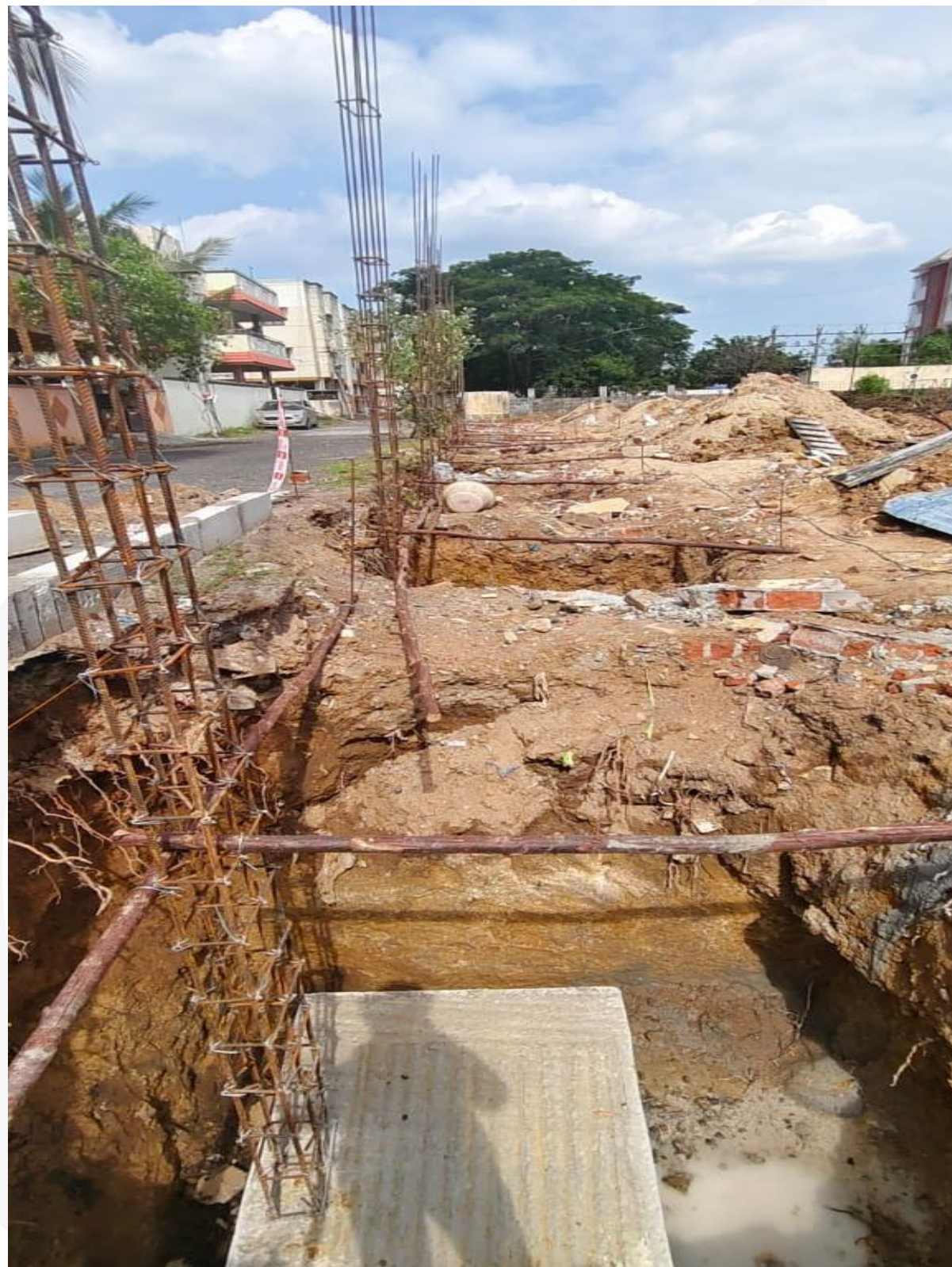
NORTH SIDE COMPOUND WALL FOOTING CONCRETE WORK IN PROGRESS
