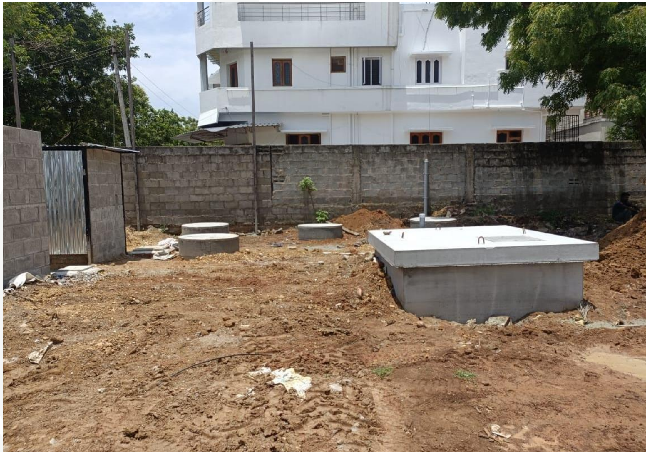
LABOUR SHED PLUMBING WORK COMPLETED
