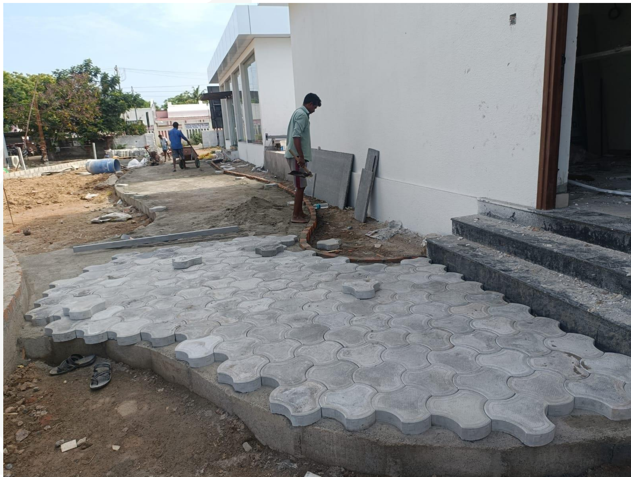
PATHWAY PAVER BLOCK LAYING WORK IN PROGRESS
